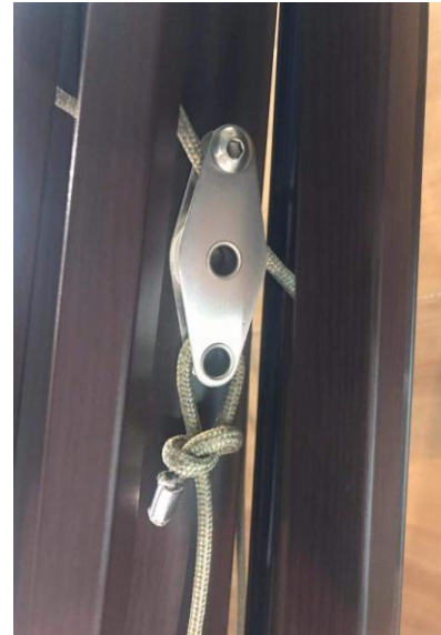
4. Go through the underside of upper pulley and tie a knot. Please note the knot is Flemish knot.
